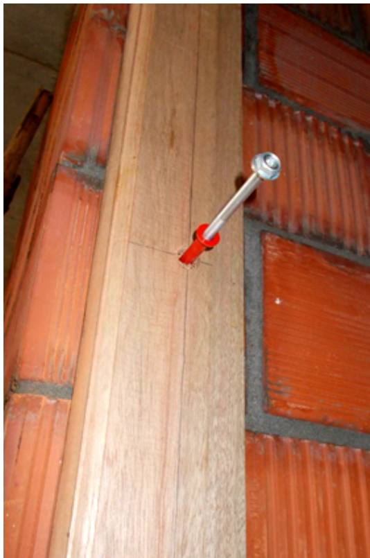
Step: 3 Install the ancor
