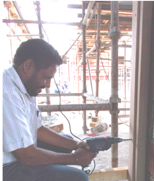
Step: 2 Drill a suitable hole as per the anchored size
