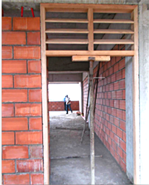
Step:1 Align the door with proper line and level
